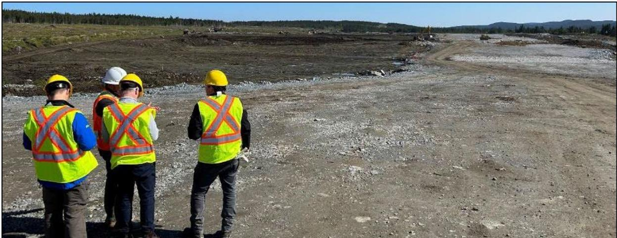
*Figure 2: "Zone 6" Rockfill placed on prepared and approved foundation for the TMF Phase 1 Dam, looking northwest. On the upstream side (top left of photograph) shows the prepared foundation without any fill material placement, August 29, 2023.*
