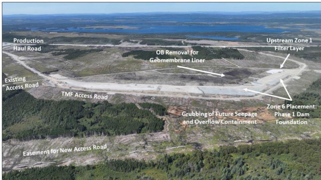
Figure 1: Overview of TMF Construction, September 2, 2023
